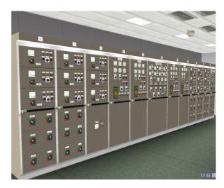
Electric Power Plant is equipped with modern Power Management System which enables automatic control of generators according to actual power demand.
